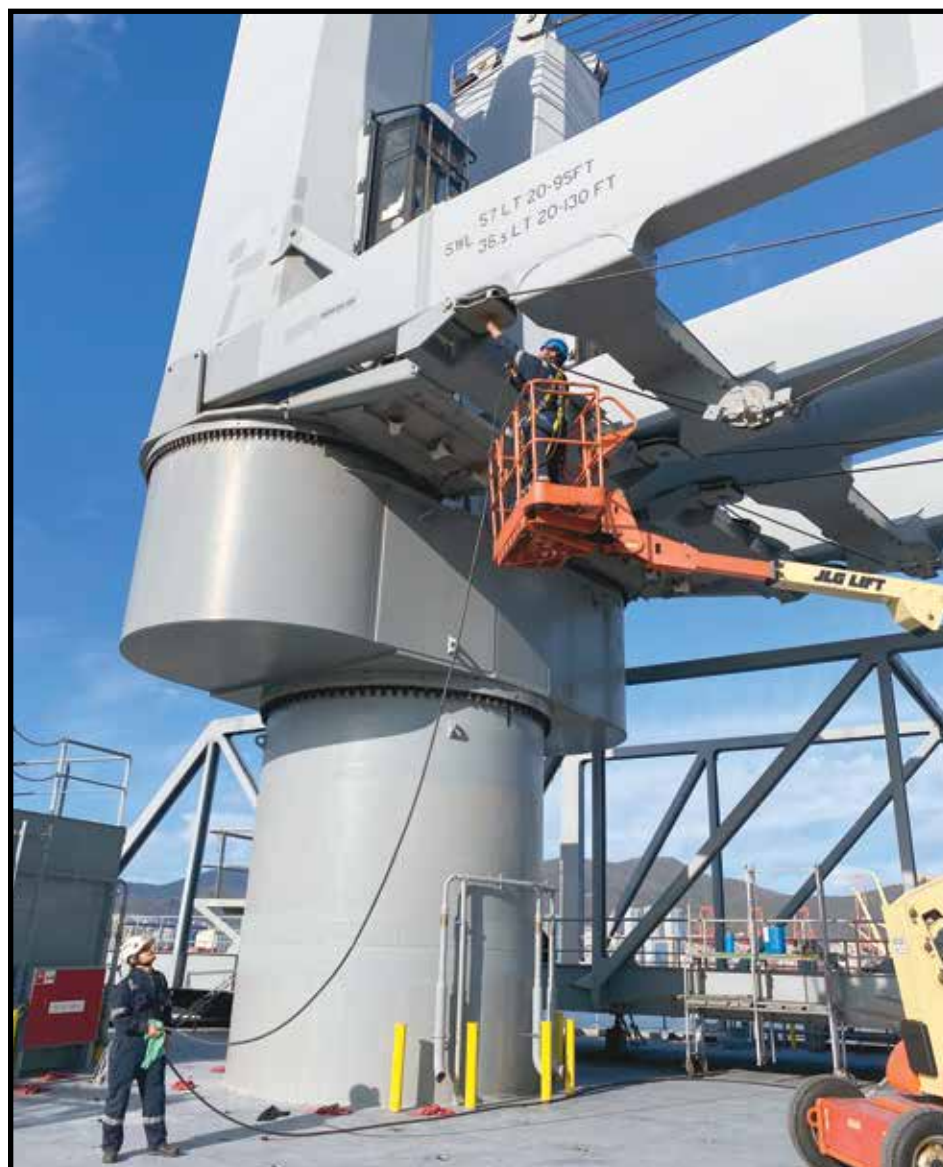
AB Isiah Montoya works aloft greasing crane block sheaves aboard USNS WATKINS. On deck AB Abdul Mohamed assists handling the grease line and serving as spotter on November 16, 2020 in Korea.
