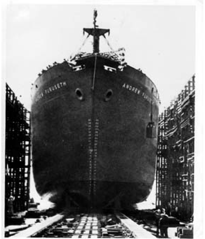
The Liberty Ship s/s Andrew Furuseth pictured above at her launching on October 8, 1942. Build at Permanente Metals Corporation Shipbuilding Division in Richmond, California in less than a month, the Furuseth was designated a War Shipping Administration Transport with a capacity of 550 men and was operated by Matson Navigation Company. During World War II the Furuseth served in the Atlantic and Mediterranean Theaters. In 1947 she was sold to Norwegian interests and was renamed the Essi. In 1959 she was sold to the Japanese and renamed the Niobe. She was scrapped in Nirao, Japan in June, 1967.
