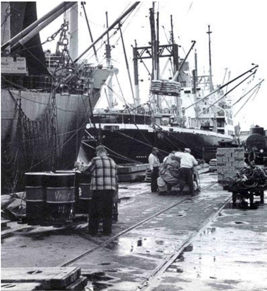
American President Lines Mariner-Class freighter President Garfield alongside in Tacoma, Washington in the 1950s. This dockside shot accurately depicts the breakbulk cargo handling gear and methods before containerization changed everything.
